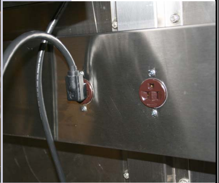
Illustration 2.D- Dual Serving Module Power Cord Plugged into Rear Distribution Panel of Flex Serving Line Cabinet
