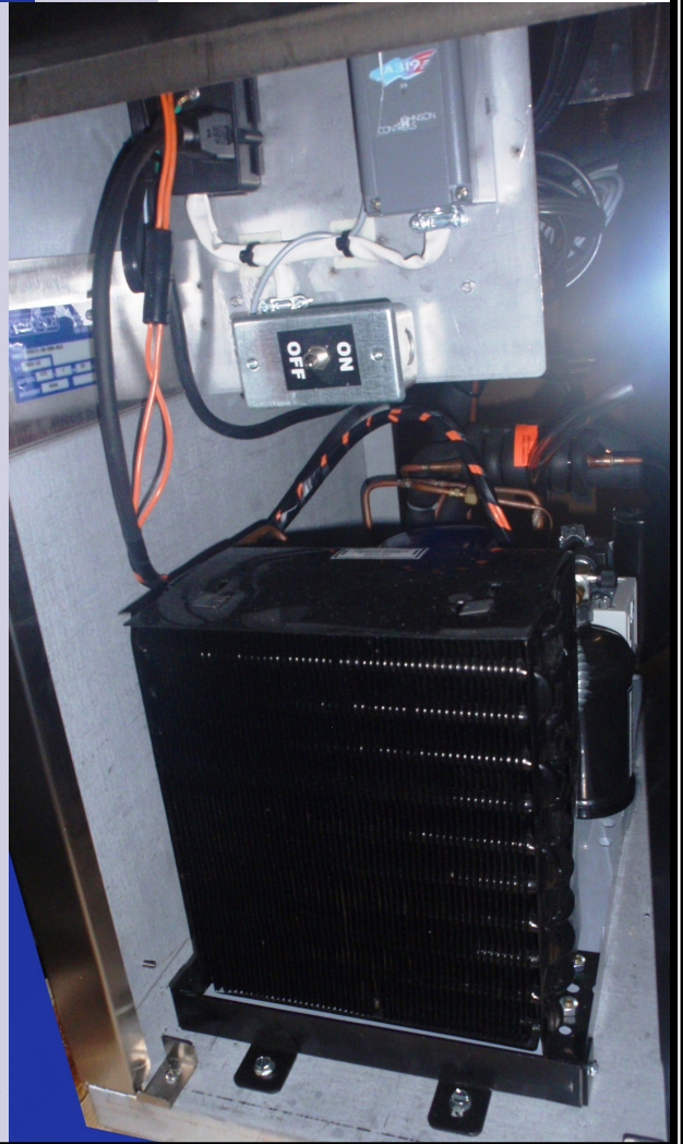
Illustration 2.B-Control Panel & Condensing Unit Assemblies
